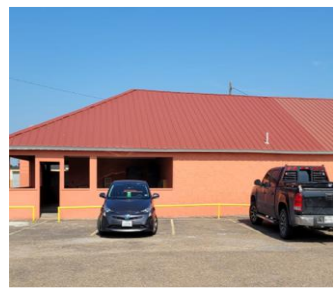
Opened back of building
