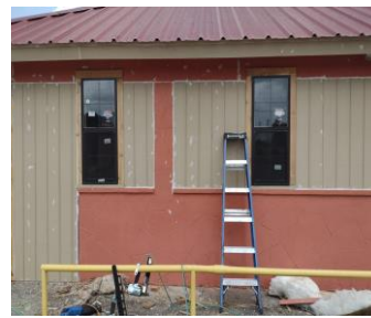
Enclosed back of building
